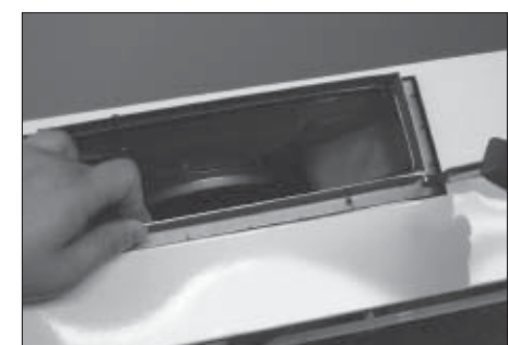
6. Mount starting collar (provided) at rear discharge.
