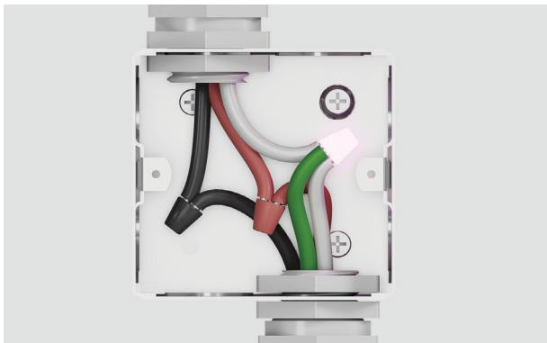
1. Connect the factory-taped green and white oven wires to the neutral (white) wire in the junction box.
