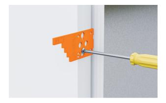
7. Slot the gauges onto the door screws. Push the gauges down to lock into position before tightening the screw to secure.
