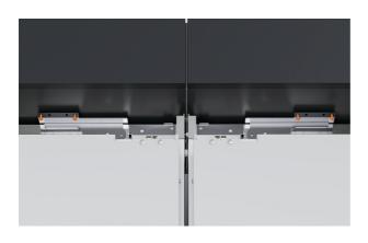
**6.** Fit the two upper brackets to the cabinetry using two 8Gx16 countersunk screws on each side.
