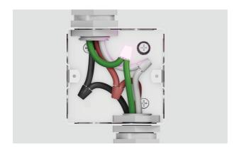
5. Connect the green grounding oven cable wire to the (green) grounding wire in the junction box. Do not connect the green grounding wire to the neutral (white) wire in junction box.
