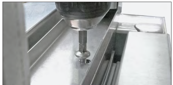
FIG. 10. Remove the screws from the metal channel.
