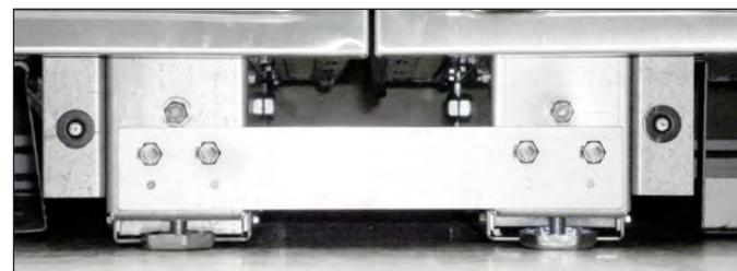
FIG. 18. Installed joining bracket.
