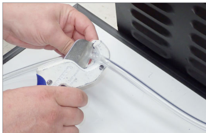
FIG. 3. Cut the drain line with tubing cutters.
