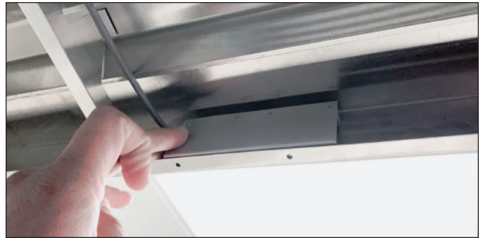
FIG. 3. Locate the reed switch in the bottom of the rainshield.
